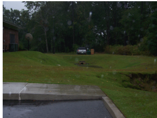
Earthen Pond with Structural Wall
