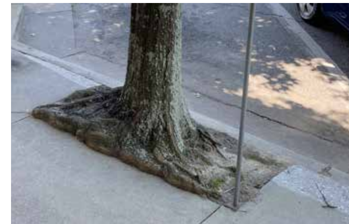
For tree plantings such as this one in the historic downtown district where the tree well is too small, the city can install structural cells that provide more soil volume for larger and healthier trees while allowing for high traffic volume.
